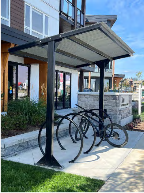
Figure 5.4: Weather-Protected Structure for Bicycle Stall
