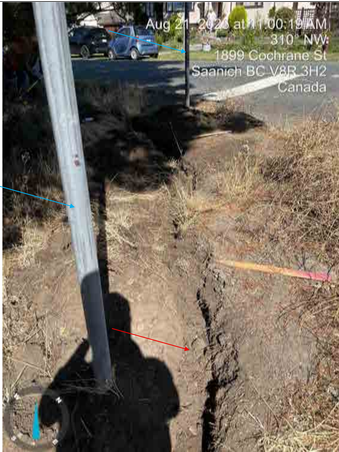
Photograph 2: Area of hand-dug exploratory excavation along the backside of the proposed sidewalk (wooden stake) on the northeastern side of tree 2249 (Corner of Dean Avenue and Cochrane Street). Larger ~12-14cm root (red arrow indicates approximately location, it is not visible in this photo) located near the base of existing street sign “no parking”. To our understanding the let down area of the sidewalk to the road grade is between the no parking street sign and the stop sign (blue arrows).
