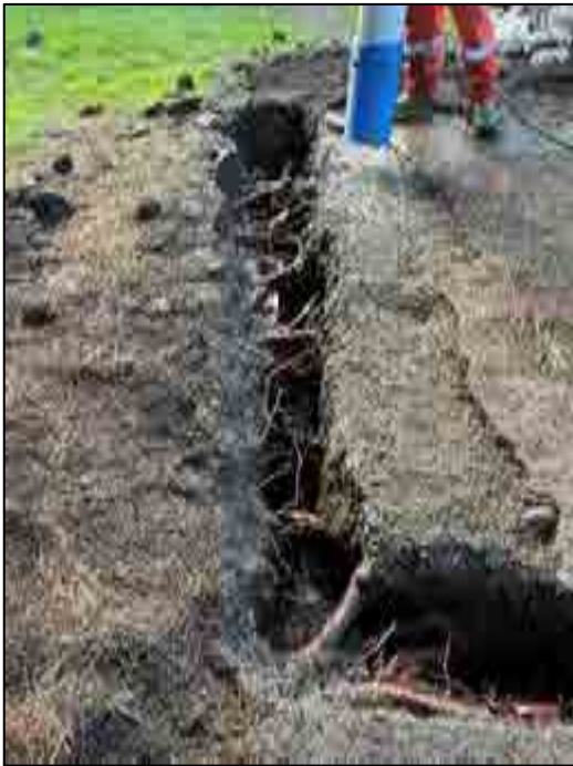
Photographs 5 & 6: Continuation of rooting structures encountered during southwest exploratory excavation. Some of these rooting structures will require pruning during the over-excavation for the building footprint.
