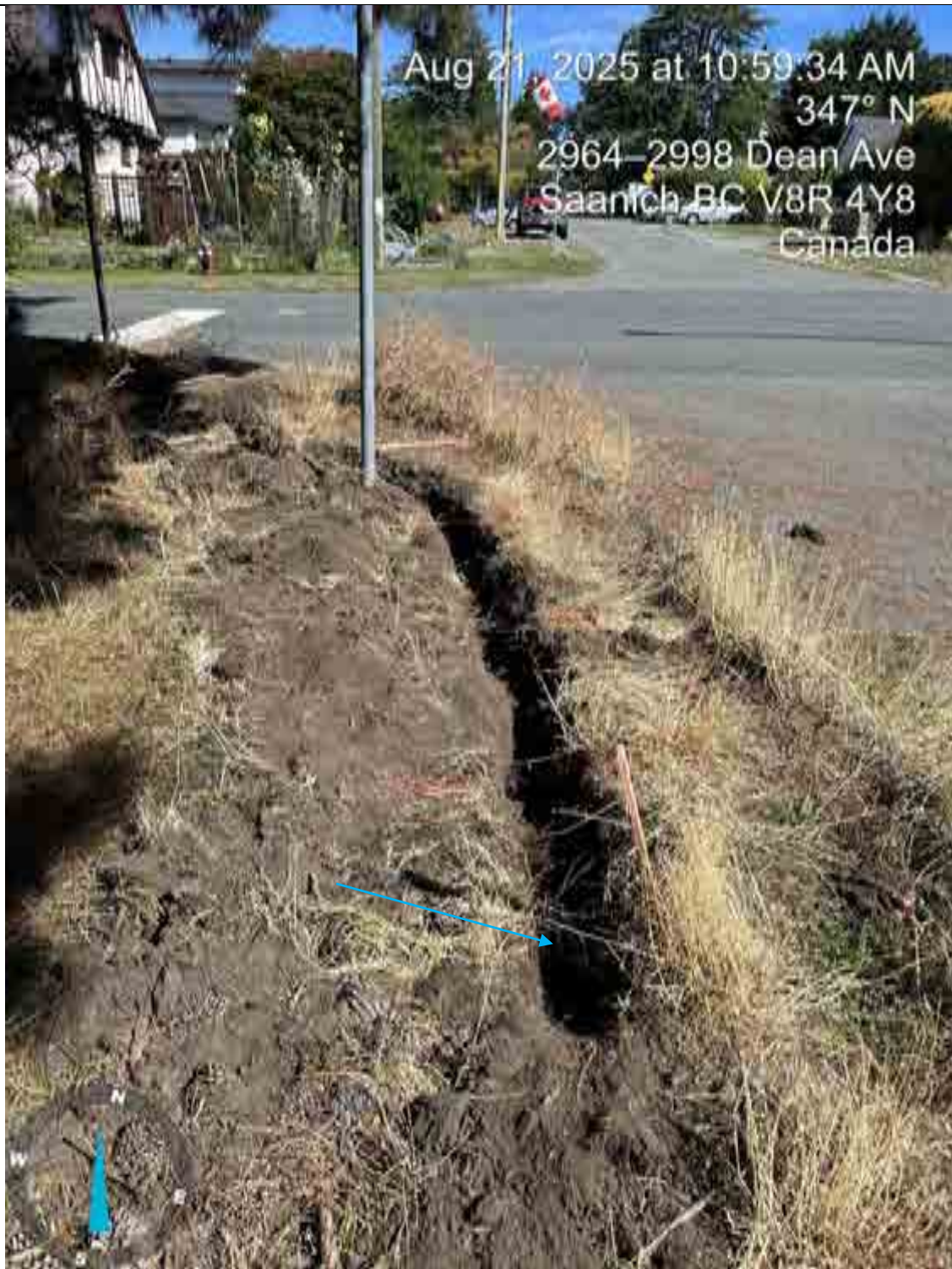
Photograph 1: Area of hand-dug exploratory excavation along the backside of the proposed sidewalk (wooden stake – red arrow) on the east side of tree 2249 (Dean Avenue frontage). Larger rooting structures previously encountered (blue arrow, difficult to see) were found to be 20-25cm below the existing boulevard grade.
