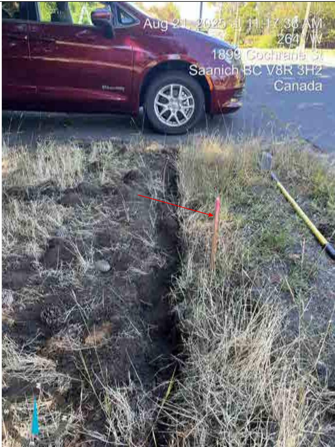
Photograph 6: Area of hand-dug exploratory excavation along the backside of the proposed sidewalk (wooden stake – red arrow) on the north side of tree 2249.
