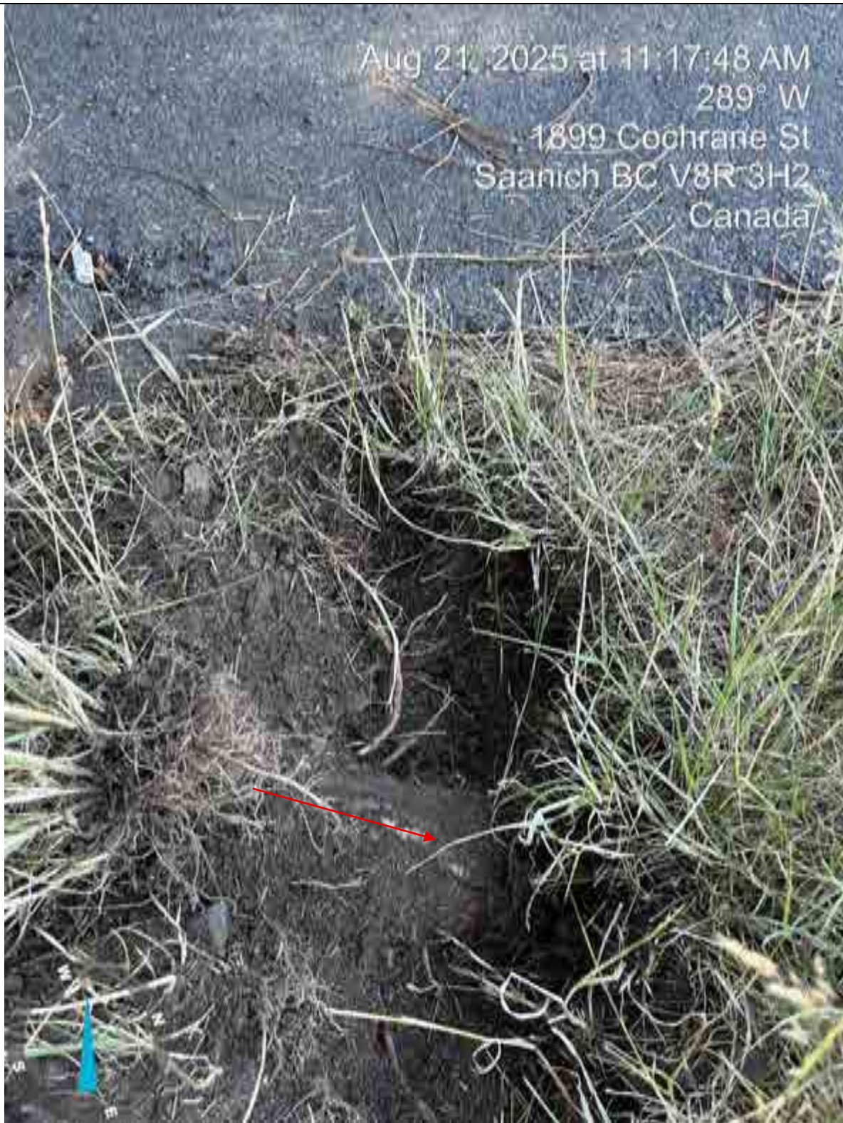
Photograph 7: 1x6cm root (red arrow) exposed just east of the existing driveway during the had-dug exploratory excavation on the north side of tree 2249 along the Cochrane Street frontage.
