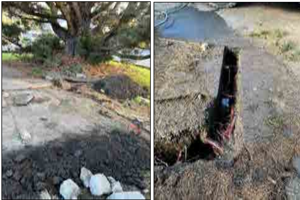
Photographs 3 & 4: Area on the southwest side of the tree was marked out for the exploratory excavation ( left photo ). Rooting structures encountered during the southwest hydro-vac excavation ( right photo ). These structures will have to be pruned during the over-excavation for the building footprint.
