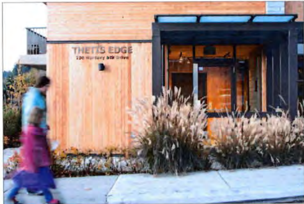
Prominent main building entrance provided from the public street.
