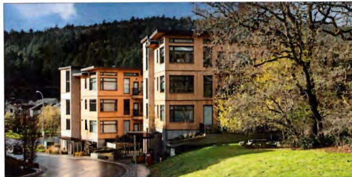
Building elevations fronting the park with significant grade difference.
