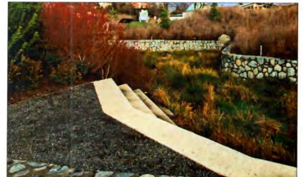
Terraced rear yard with retaining walls.
