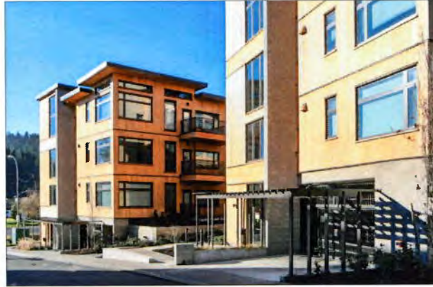
Vehicle access from entry lane.
