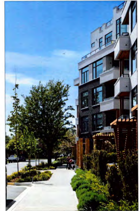
Private outdoor spaces and landscape buffers facing the street.
