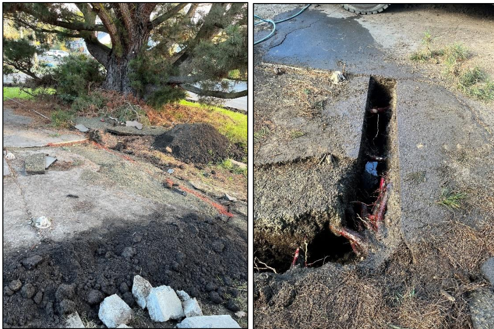
Photographs 3 & 4: Area on the southwest side of the tree was marked out for the exploratory excavation ( left photo ). Rooting structures encountered during the southwest hydro-vac excavation ( right photo ).
