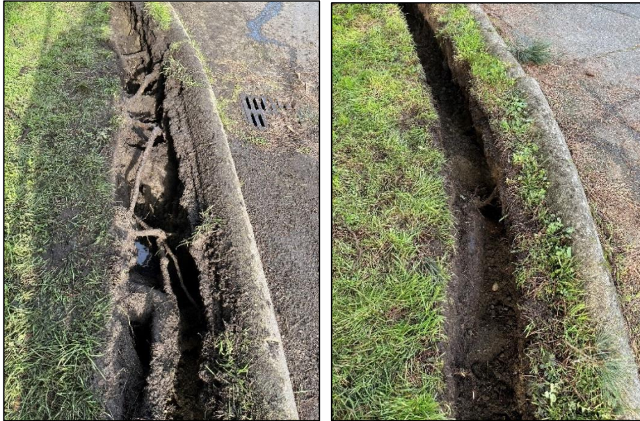
Photographs 1 & 2: Larger rooting structures (~10-20cm in diameter) were exposed approximately 6.5 east of tree 2249 near the existing catch basin on Dean Avenue ( left photo ). More larger rooting structures encountered ~6m northeast from the root collar of tree 2249 ( right photo ).
