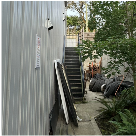
PHOTO OF EXISTING STAIR ON WORKSHOP NORTH ELEVATION
